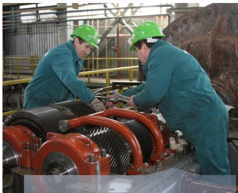
Dynamic Equipment Installing & Maintenance Department
