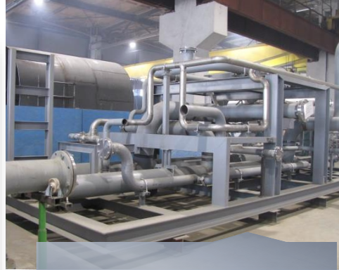
Fabrication steel structures
